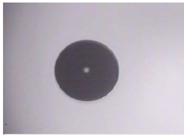
Clean fiber optic jumper
